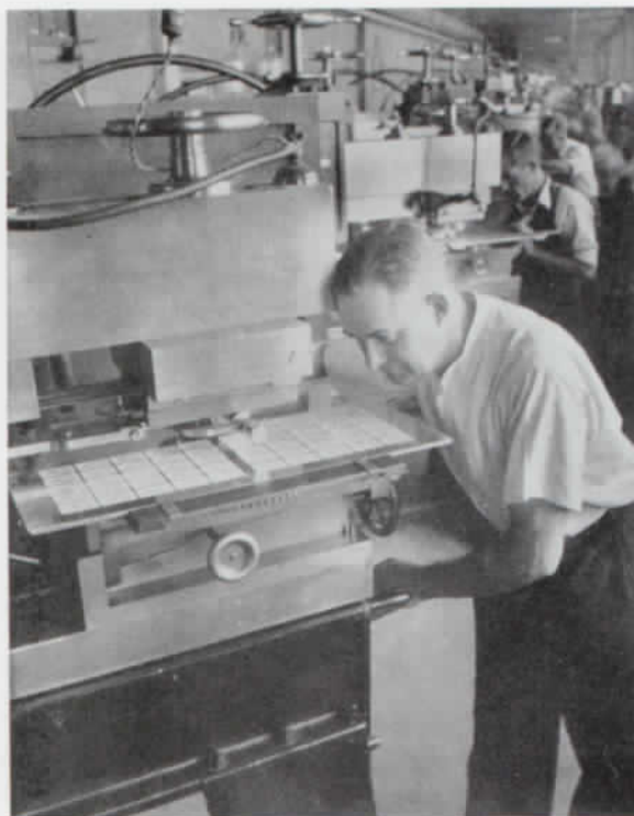
Figure 6. Transfer press circa 1930 showing partially entered plate
